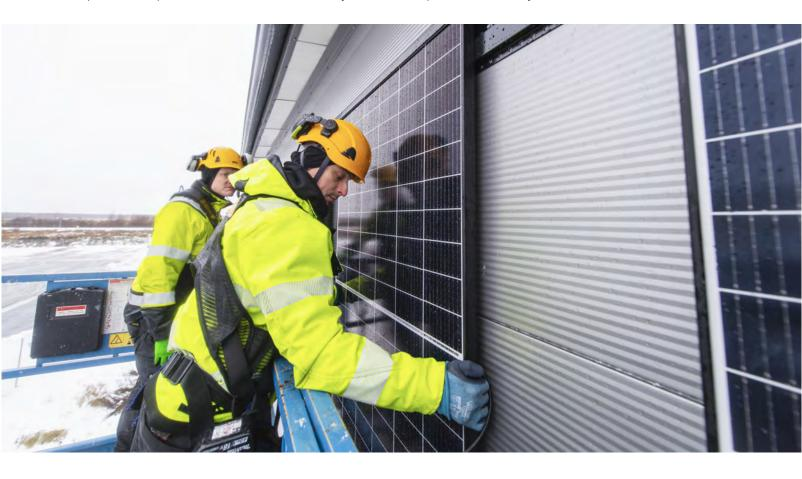
If the panels must nevertheless be installed horizontally -- for example to take advantage of usable space -- please note that a larger mounting system and more attachment accessories will be necessary.
