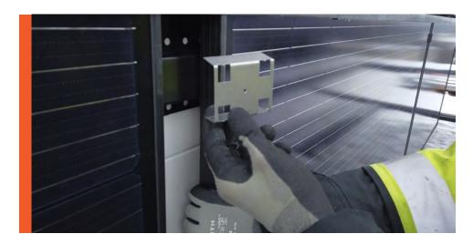
Between the solar panels, one earthing plate is installed under the upper intermediate clamp.
