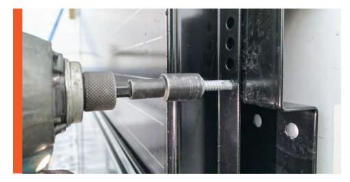
The end profiles are attached using four 6.3 x 19 mm screws with RUSPERT coating.
