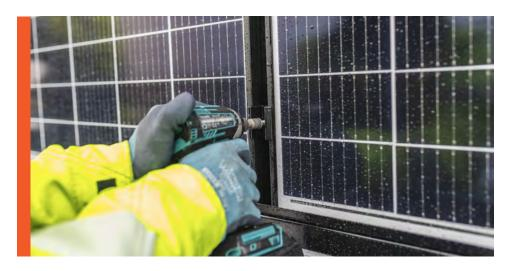
The intermediate clamp is attached using one 6.3 x 38 mm screw with RUSPERT coating.
